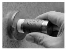
**2.** Screw the valve into the female thread by hand until firm\*.
