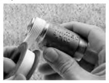
I. Apply PTFE tape or approved sealant to the thread ensuring a sufficient amount is applied to guarantee a watertight seal.
