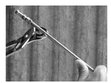
4. Where necessary bend the lever arm to adjust the water level. This can be done by removing the lever arm assembly by first straightening the tabs on the end of the pivot pin with a pair of pliers then slide it out.
