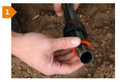
Cut the pipe square and place the nut and grip ring on to the pipe.
