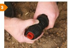
Position the insert in the body of the fitting, position the grip ring and nut and tighten by
