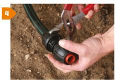
Tighten the nut with a wrench.
