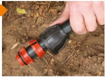
Tap the insert fully into the pipe.
