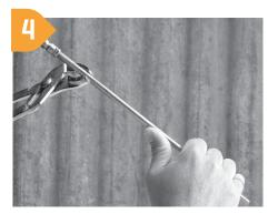
Where necessary bend the lever arm to adjust the water level. This can be done by removing the lever arm assembly by first straightening the tabs on the end of the pivot pin with a pair of pliers then slide it out.
