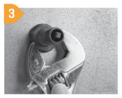
Using a pipe wrench or multigrips on the hex of the valve, screw it into the female thread until tight. Where necessary ensure the female thread is held stationary to avoid it from moving.
