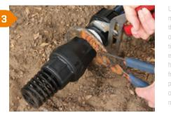
Using a pipe wrench or multi-grips further screw the non-return/foot valve onto the male thread until tight. Where necessary ensure the male thread is held stationary to avoid it from moving. Do not use pipe wrench or multi-grips on the body of the non-return/ foot valve.
