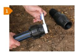
Apply PTFE tape or approved sealant to the male thread the non-return/foot valveis to be screwed onto. Sufficient tape needs to be applied to ensure a water tight seal.
