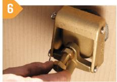
Adjust the float level by screwing the adjusting bolt in [clockwise] or out [counter clockwise] of the cam. Screwing the bolt out lifts the water level, screwing it in lowers the water level. Once the desired level is found ensure the lock nut is tightened to stop the adjusting bolt from moving. Note if valve weeps, tighten adjusting bolt an additional half turn to ensure shut off is achieved.
