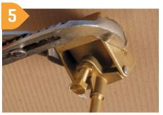
A Tighten the body of the valve using a pair of multigrips or a spanner.
