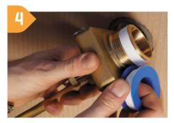
Apply PTFE thread tape to the thread and screw the valve into the tank/trough outlet.
