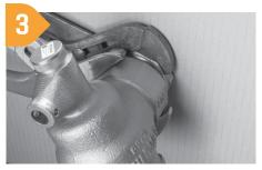
Using a pipe wrench or multigrips on the hex of the valve, screw it into the female thread until tight. Where necessary ensure the female thread is held stationary to avoid it from moving.
