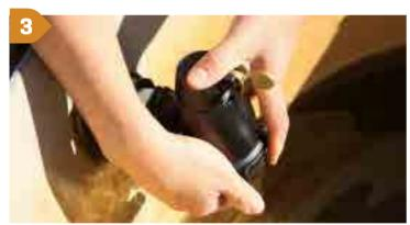
Screw in the float valve body by hand only until firm and in the vertical position.
