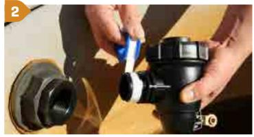
Apply PTFE thread tape or approved sealant to the thread ensuring enough is applied to ensure a water tight seal.
