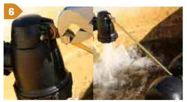
Insert the bolt and tighten with a shifter. The bolt can be loosened to make adjustments to the water level. Float valve is now fully installed.
