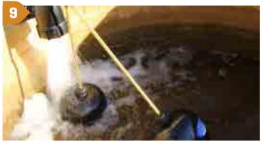
Float valve is now fully installed.
