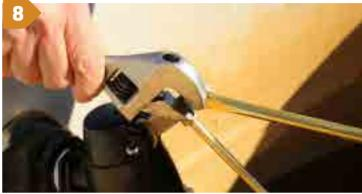
Insert the bolt and tighten with a shifter. The bolt can be loosened to make adjustments to the water level.
