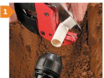
The fitting is pre-assembled and ready to use. Cut pipe square and to length using the flange on the central body as a guide. Ensure the end of connecting pipe is undamaged and clean.
