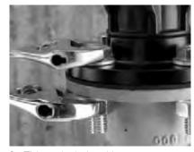
**3.** Tighten the bolts with a spanner ensuring the bolts are torqued up correctly in an appropriate sequence.
