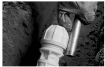
3. Pipe insertion: To ensure adequate insertion depth, witness mark the pipe to the flange on the fitting. Then insert pipe to the correct depth.
