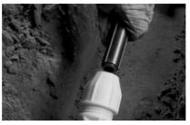
2. Ready to use position: The fitting is pre-assembled and ready to use, however always ensure the nut is backed off with 3 threads showing to allow pipe to pass freely.
