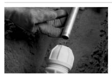
I. Cut pipe to length: Cut pipe square and to length using the flange on the central body as a guide. Ensure end of connecting pipe is undamaged and clean.
