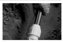
3. Pipe insertion: Gently insert the pipe until the first point of resistance is felt.
