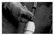
I. Preparation of pipe end. Cut Pipe Square. There is no need to chamfer the
