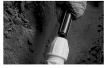
6. Disassembly: To disassemble the fitting, simply loosen the nut using a wrench until 3 threads are showing. Pipe will be released and can be pulled out of the fitting.
