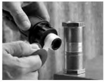
**I.** Apply PTFE tape or approved sealant to the thread ensuring sufficient is applied to ensure a watertight seal.
