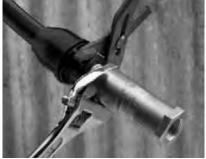
**3.** Using a pipe wrench or multigrips on the hex end of the valve, screw it into the male thread until tight. Where necessary ensure the male thread is held stationary to avoid it from moving.
