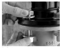
**2.** Fit the correct size and length bolts to each hole in the flange and hand tighten them.
