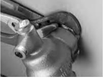
**3.** Using a pipe wrench or multigrips on the hex of the valve, screw it into the female thread until tight. Where necessary ensure the female thread is held stationary to avoid it from moving.
