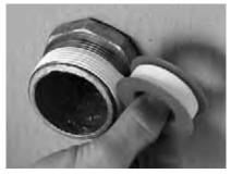
Apply PTFE tape or approved sealant to the inlet thread ensuring sufficient is applied to ensure a watertight seal.
