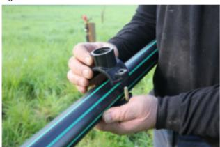
3. Assemble the saddle halves in the desired location on the Rural poly pipe.
