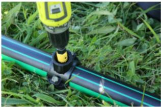
5. Drill a hole using the correctly sized drill bit taking care not to damage the seal or thread.
