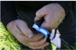
6. Connect the desired threaded fitting to the outlet using PTFE tape.
