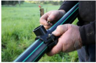
4. Thread each nut onto the bolt until firm and then complete tightening with a spanner.
