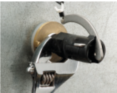
3. Using a pipe wrench or multigrips on the body of the valve screw it into the female thread until tight. Where necessary ensure the female thread is held stationary to avoid it from moving.
