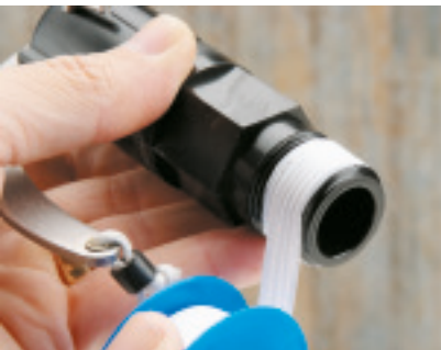
1. Apply PTFE tape or approved sealant to the thread ensuring sufficient is applied to ensure a watertight seal.
