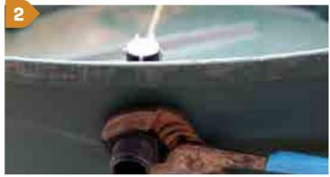
Screw the back nut on by hand and then tighten nut using multi-grips or adjustable wrench.
