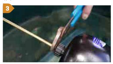
Attach the float to the threaded end of lever and tighten the locking nut with multi-grips or adjustable wrench.
