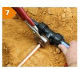
7. The nut should be tightened firmly with a wrench.
