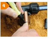
4. Cut copper pipe square. The fitting is preassembled and ready to use. Mark the depth of copper using pipe stop marking or body f lange as a visual indicator.
